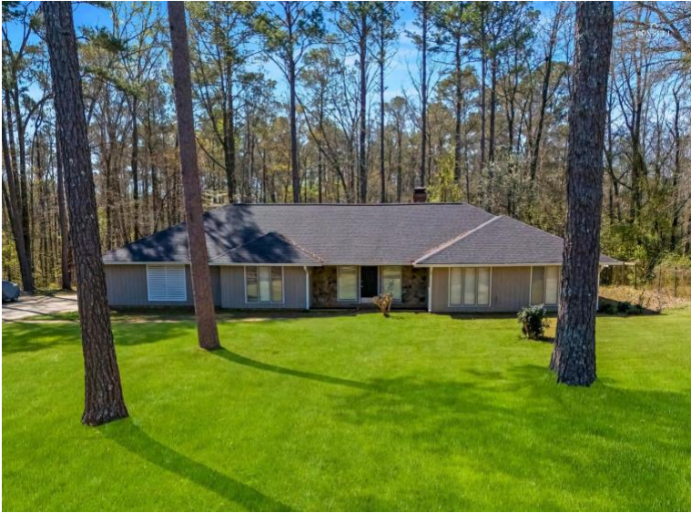
Existing ±2,700 SF residence — usable for interim income or an on-site sales/leasing office during entitlement.
