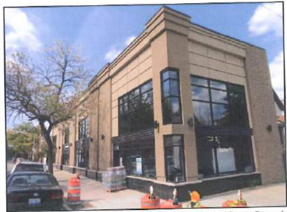
The 25th and Millard Street Offices of the Chamber Provides an Example of New Development along 25th Street.
