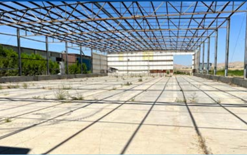
Washington Street E- Concrete Pad
