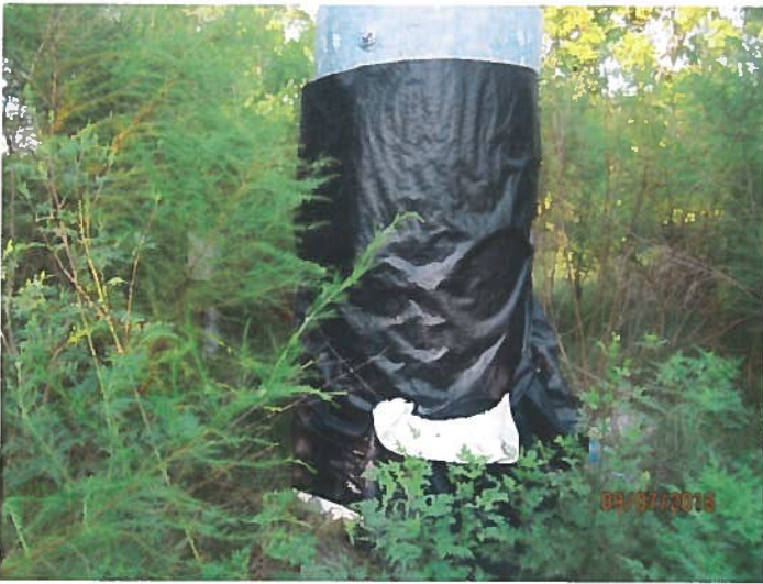
Well pump pressure tank
