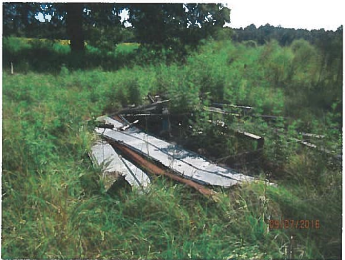
Tin and wood debris from old shed
