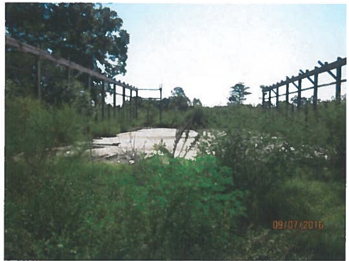
Concrete pad of former storage building
