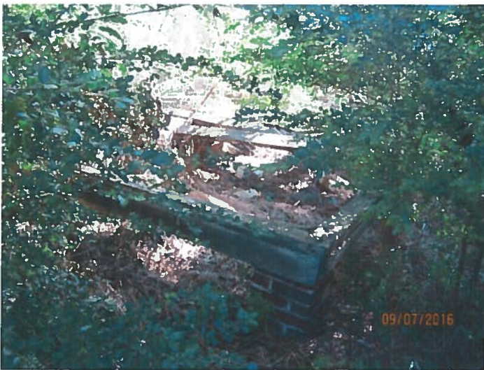
Brick pier from former home
