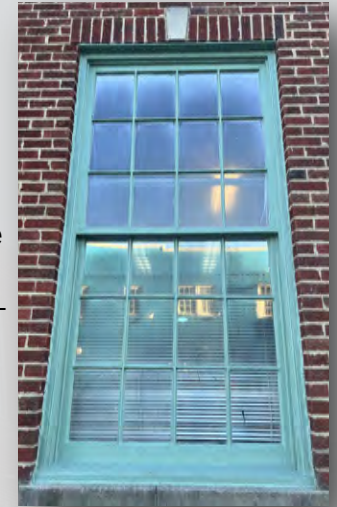
12 over 12 wood window on E. Howell side.
