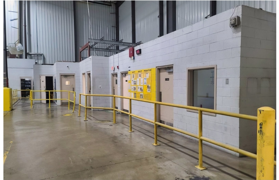
Entrance/Office Area/Restrooms/Storage Closets
