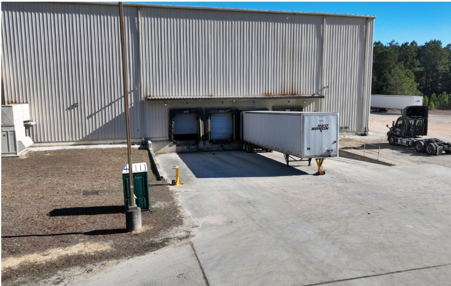
Four Loading Dock Doors Exterior
