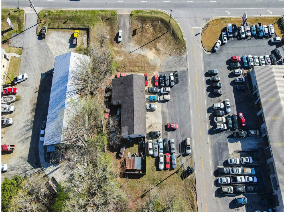
Overhead photo-Grayson Hwy
