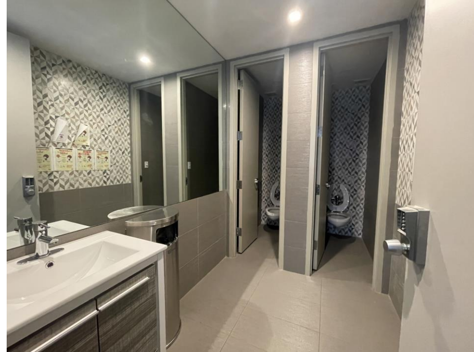
Newly Renovated Bathrooms
