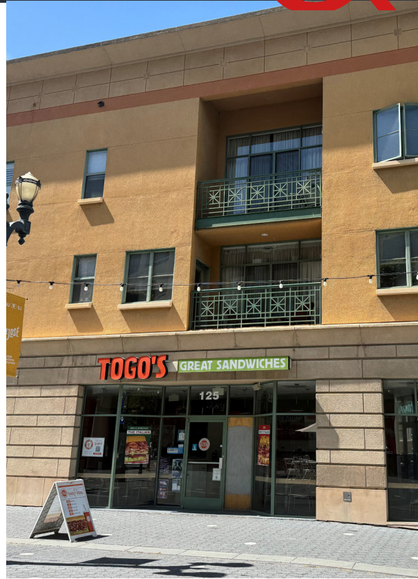
Fomer Togos Restaurant - No Hood
