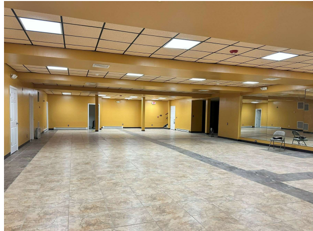
Immaculate Drop Ceilings + Flooring
