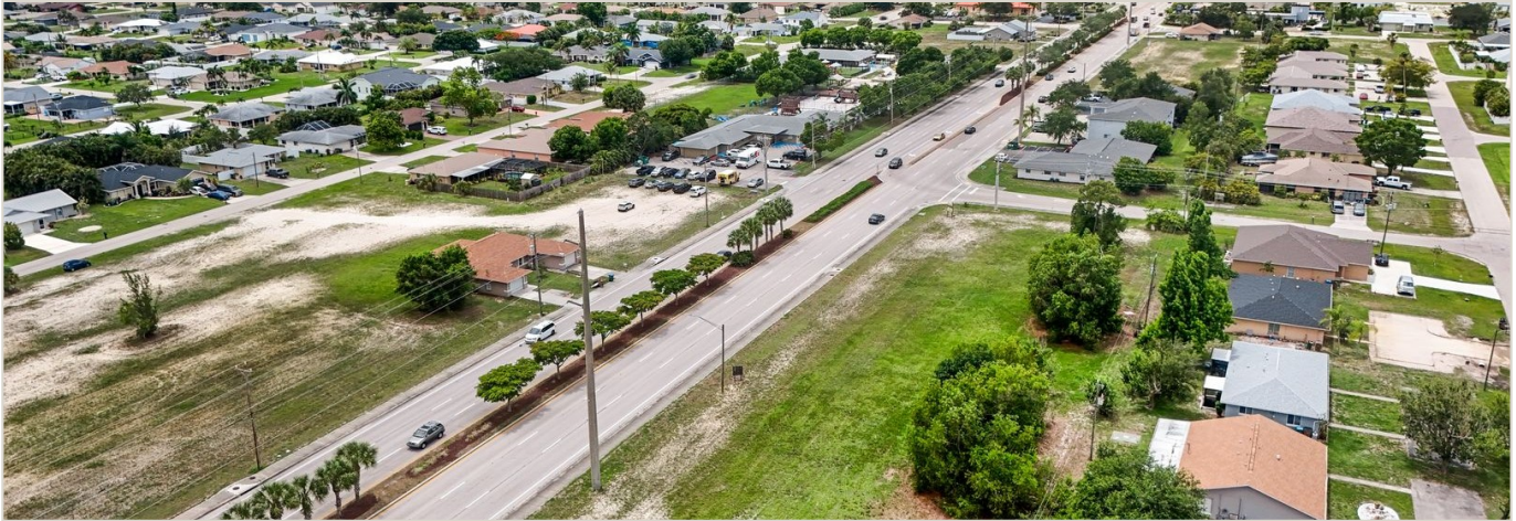
Aerial — Santa Barbara Blvd corridor & subject frontage (imagery © owner)
