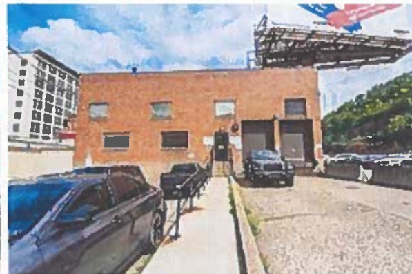
Front of Structure - This 14,000 + square feet of office and warehouse space has been leased to the same tenant for more than 20 years. There are 1st and 2nd floor offices, large conference room, bathrooms and over 8600 sq ft of warehouse space on this side.
