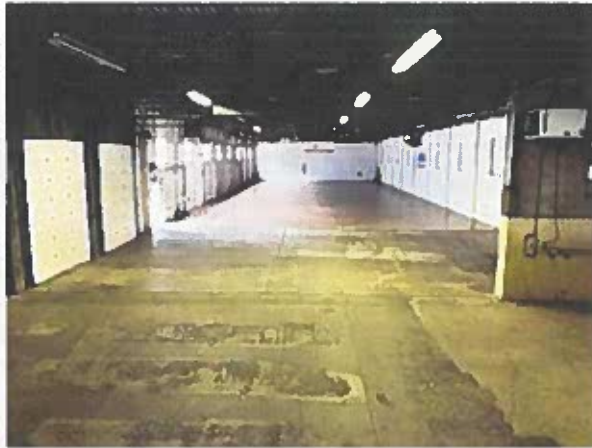
Other - View from loft area of vacant warehouse.
