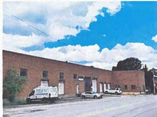
Front of Structure - View along Liberty Ave of the vacant side of 1601 Liberty Ave towards 17th St.
