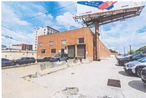
Front of Structure - View from 16th St and Liberty Ave with occupied side of the building at the end of the 16th St bridge.
