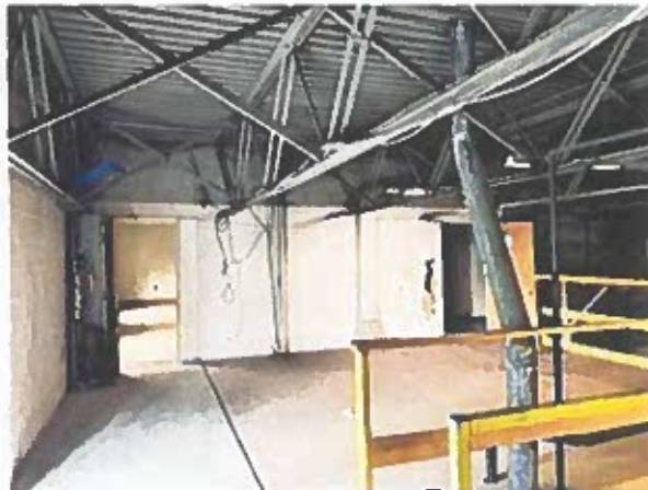
Other - 3 offices partitioned off on 2nd floor loft area.
