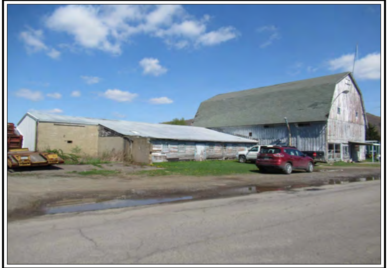
LEFT: Dry Shed - View from Main Street
