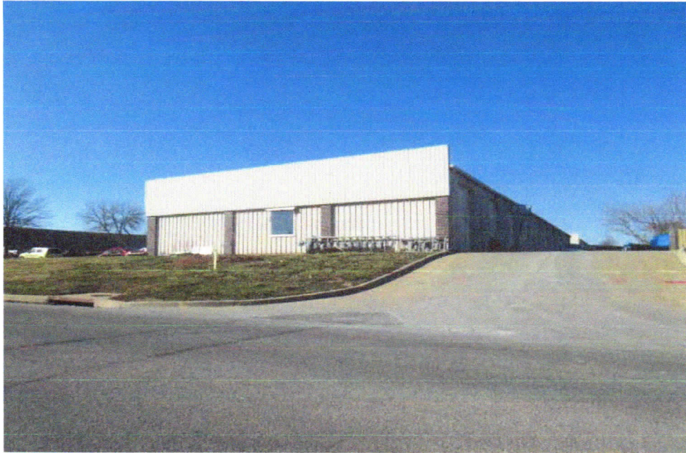
View of subject from Southeast
