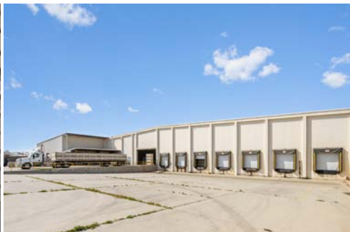
Grade Level & Dock High Loading
