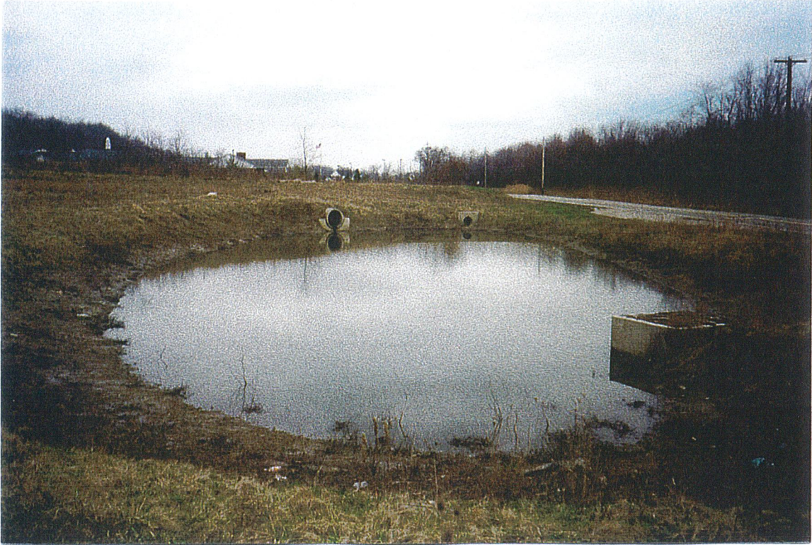
Photo 1: Looking southwest at recently constructed detention basin, from Photo Location 5.
