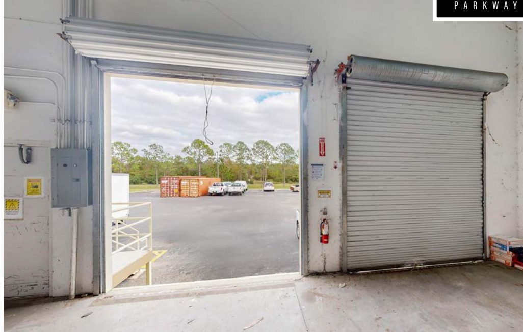
Warehouse Dock Doors
