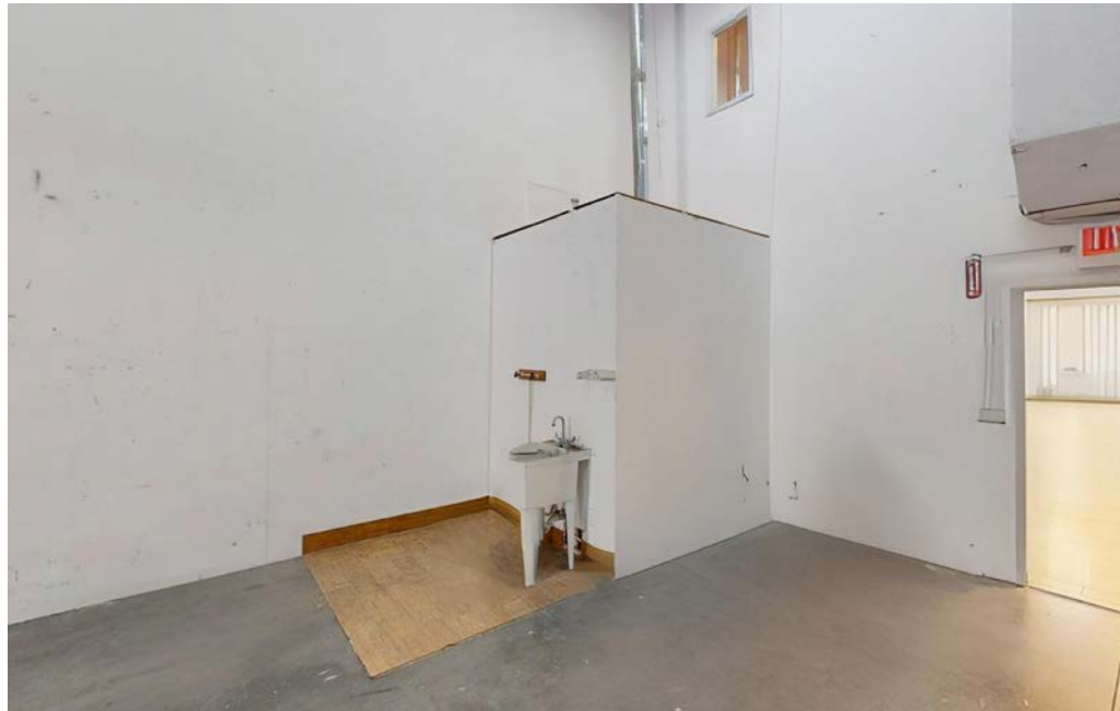
Warehouse -Utility Sink-Restroom Area
