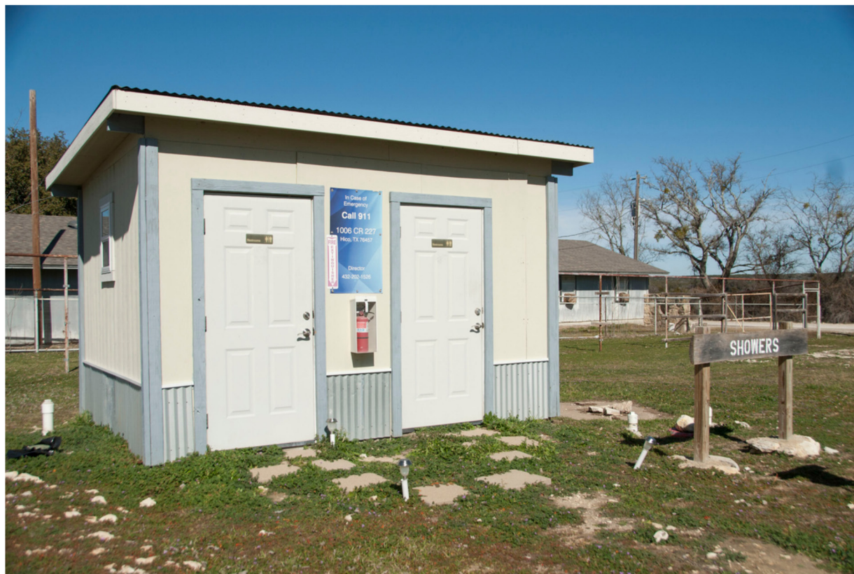
Restroom Building w/ Showers
