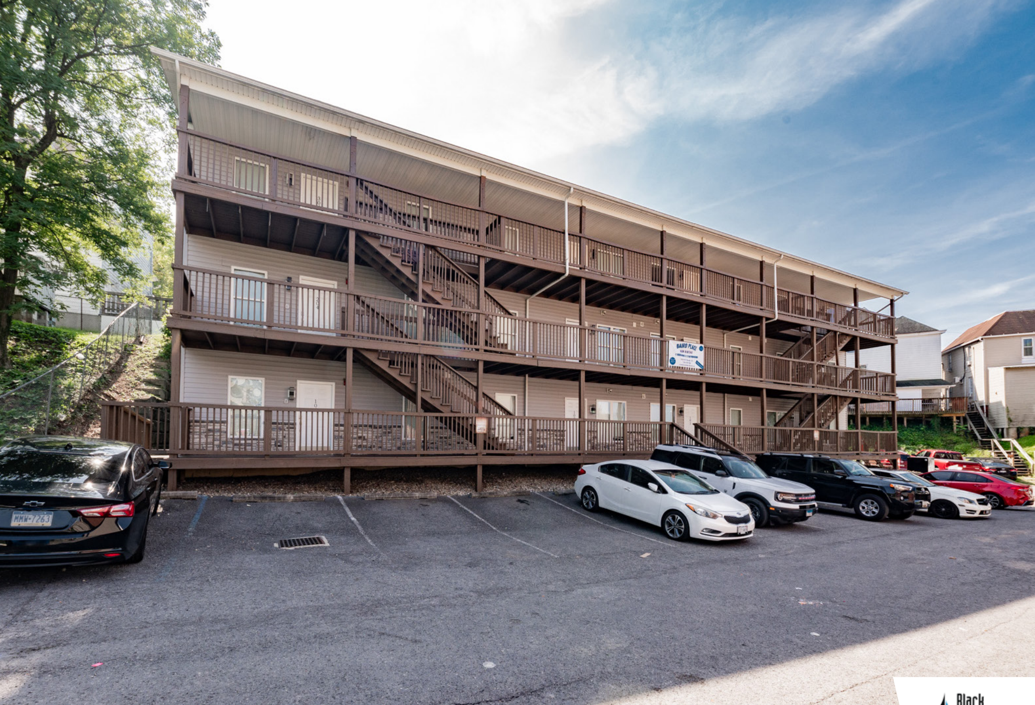
Front of Building
