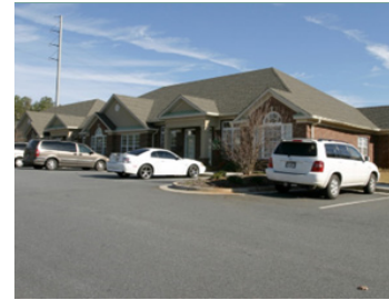
5041 Dallas Hwy – Bldg 2
