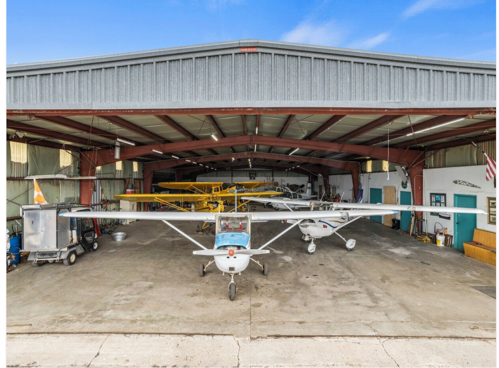
Looking into Main Hangar from outside
