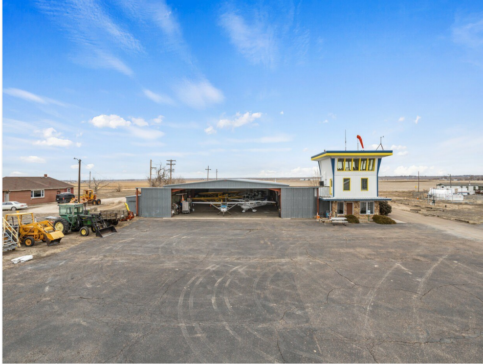
Main Hanger + Tower Exterior_Doors Open
