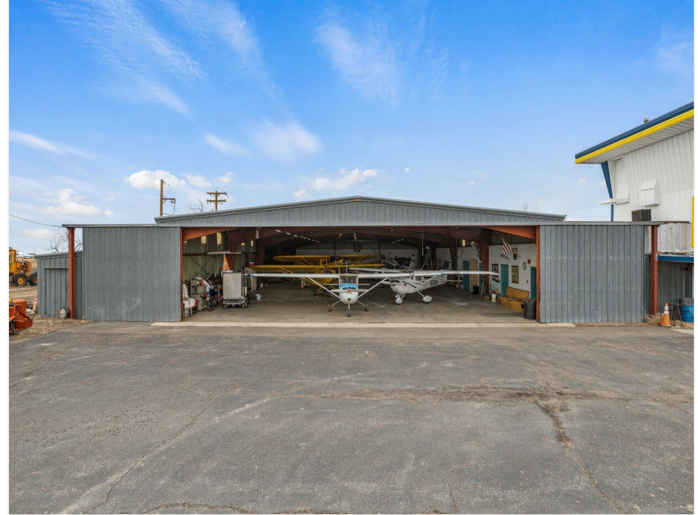
Main Hanger Looking in From Exterior
