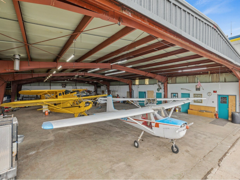
Main Hanger Interior
