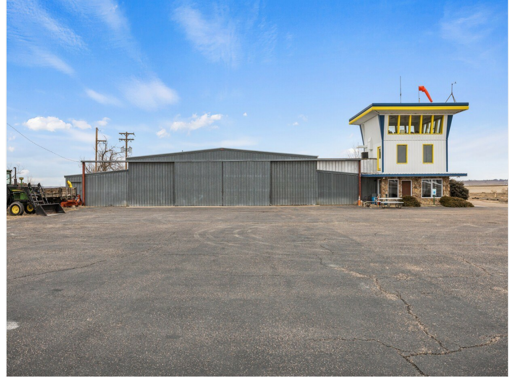
Main Hanger + Tower Exterior_Doors Closed
