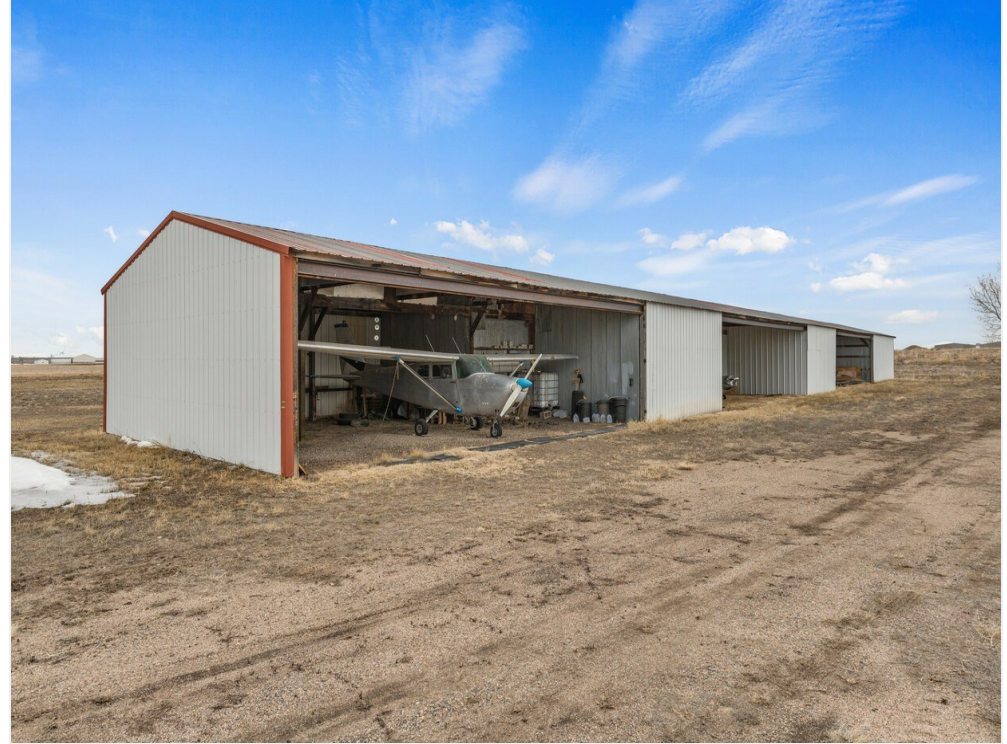
Aircraft Shelter Exterior
