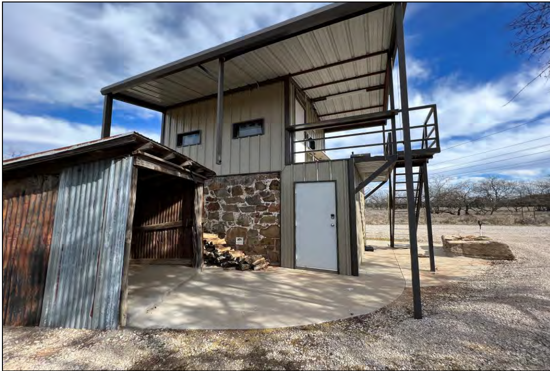
Exterior view of Building 4
