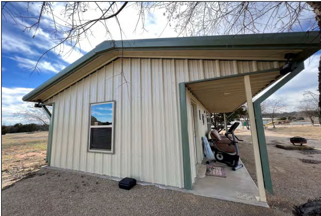
Exterior view of Building 9
