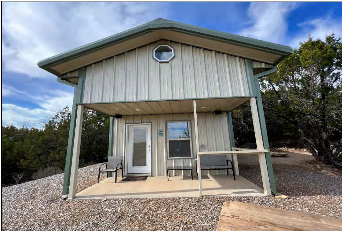
Exterior view of Building 8
