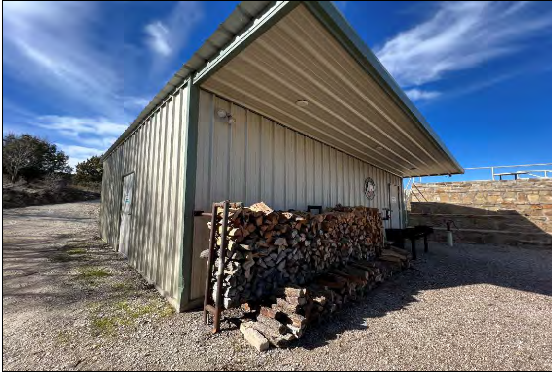
Exterior view of Building 6
