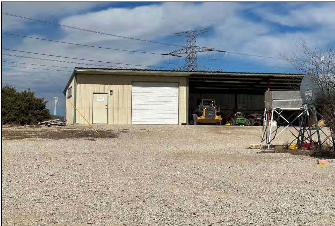
Exterior view of Building 5
