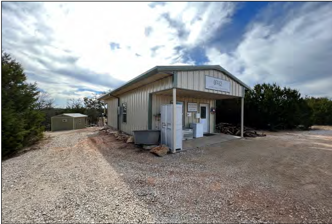
Exterior view of Building 7
