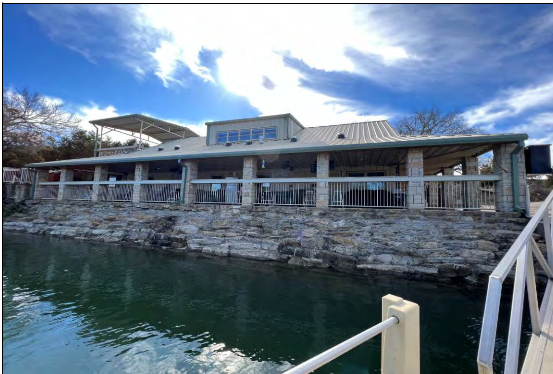
Exterior view of Building 1
