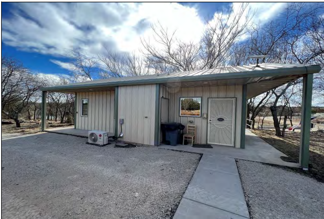
Exterior view of Building 3
