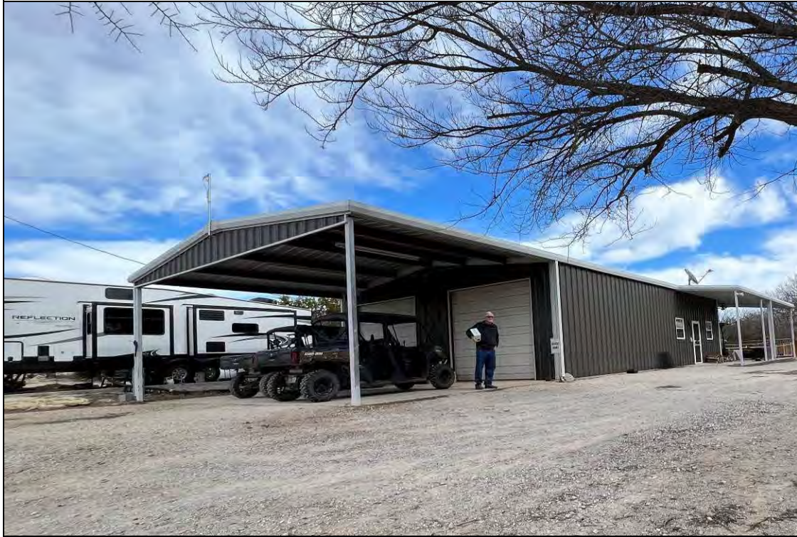
Exterior view of Building 2
