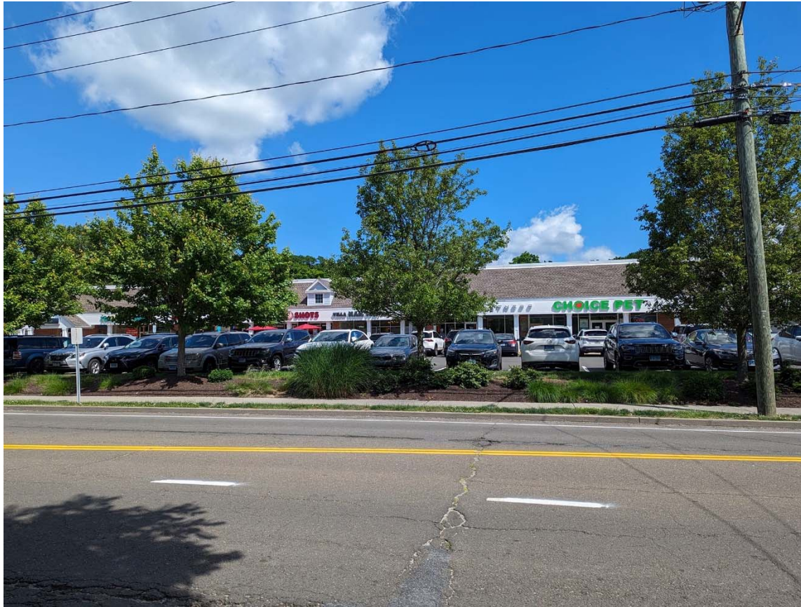
Boston Post Road (US 1) – View North – CVS Anchored Strip Center
