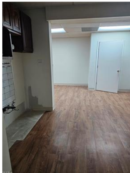
A place for a basement kitchenette to be installed.
