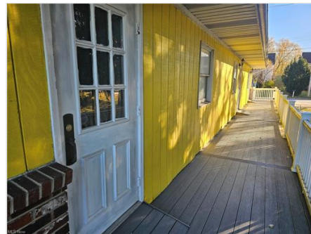
View of wooden deck
