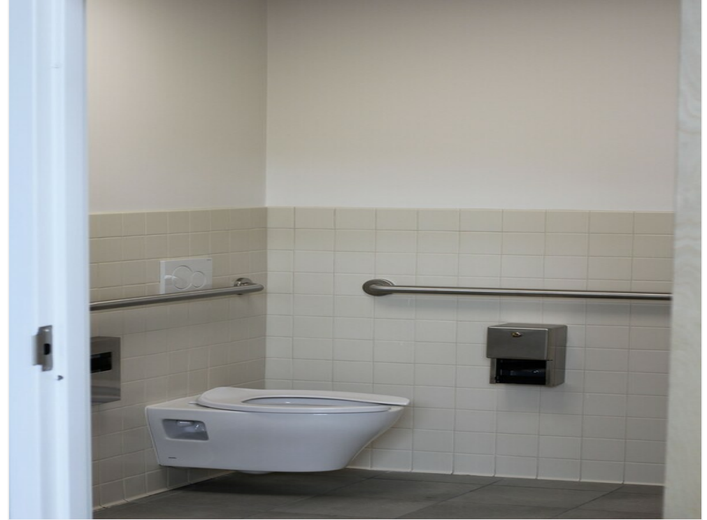
Unit B Bathroom
