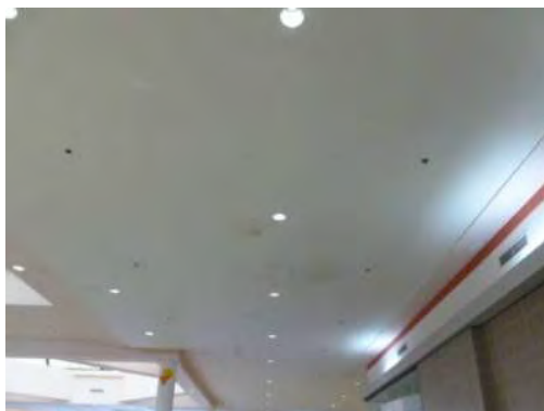
peeling and discolored ceiling finish
