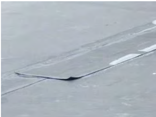
failing seam patch
