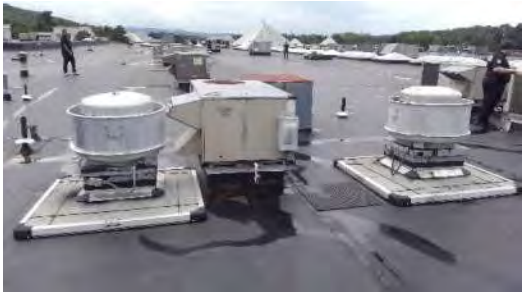
example of exhaust and plumbing vents located next to roof top unit intake
