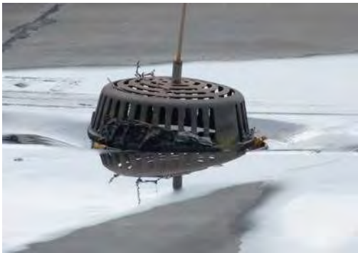
debris at drain
