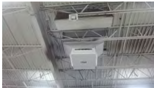
example of exposed ductwork
