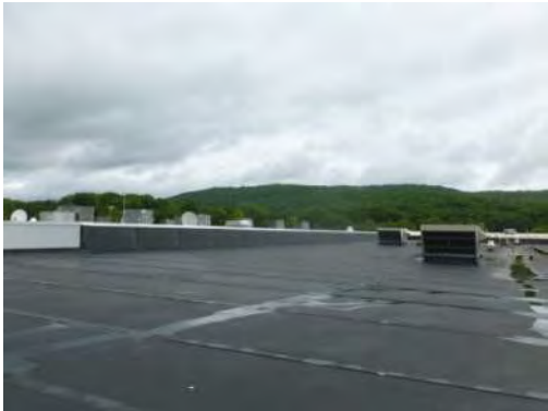
minimal ponding generally
