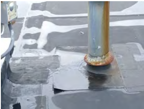
failing patch
