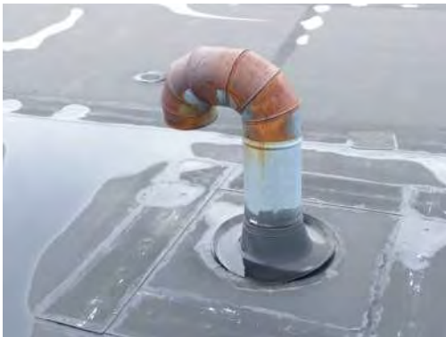
failing flashing
