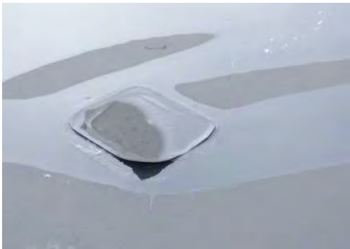
failing patch
