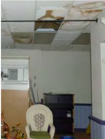
typical damage where suspended ceiling tile
