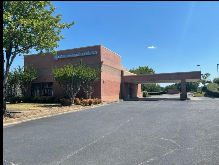
Busbee Pkwy – Eastern Elevation
