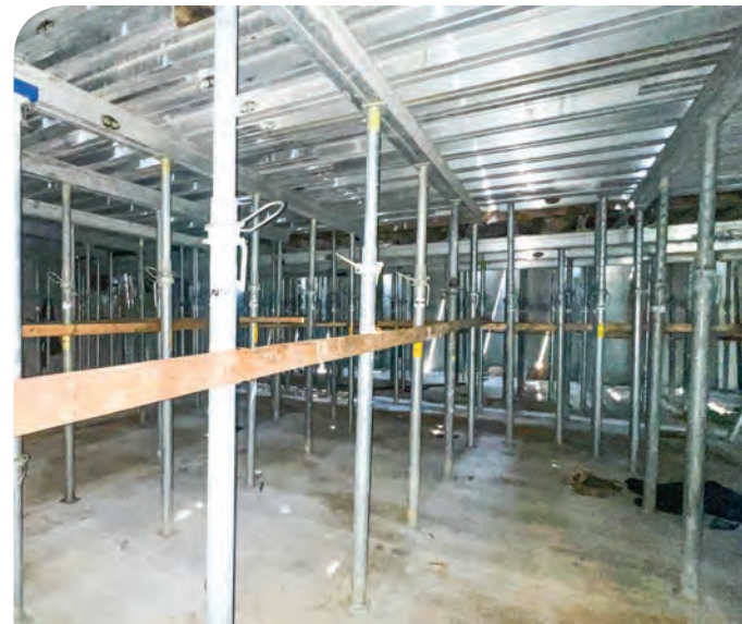
Subterranean Parking Level
