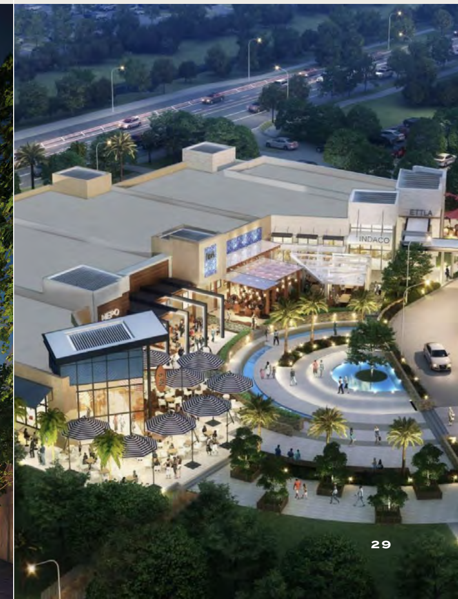
RESTAURANT ROW Orlando, FL
