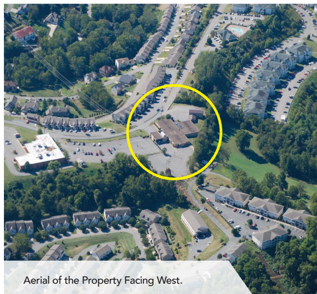
Aerial of the Property Facing North.
