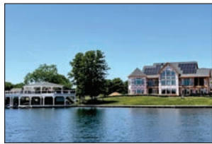
10,000 sq. ft. home under construction in the Tara Woods community of the lake by Spartan Homes.
