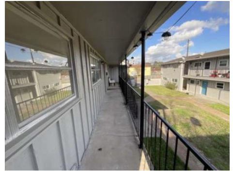
West Bldg - 2nd Floor Looking North
