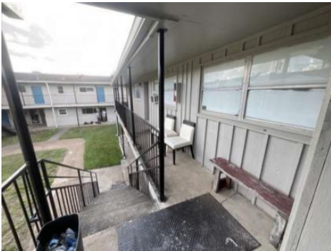
West Bldg - 2nd Floor Looking South
