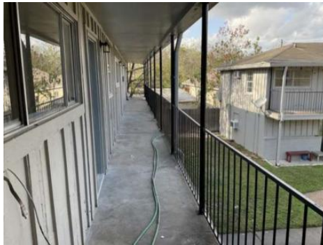
South Bldg - 2nd Floor Looking West
