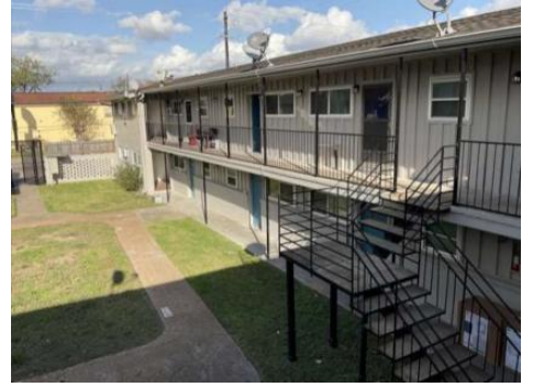
East Building Looking North
