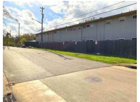
Calhoun Street along East Side of Bldg
