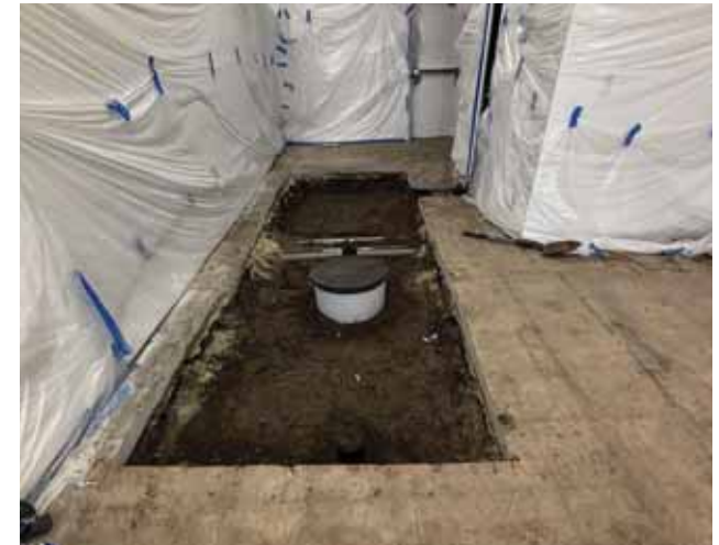
1122 Interior - Inground 40-Gallon Grease Interceptor
