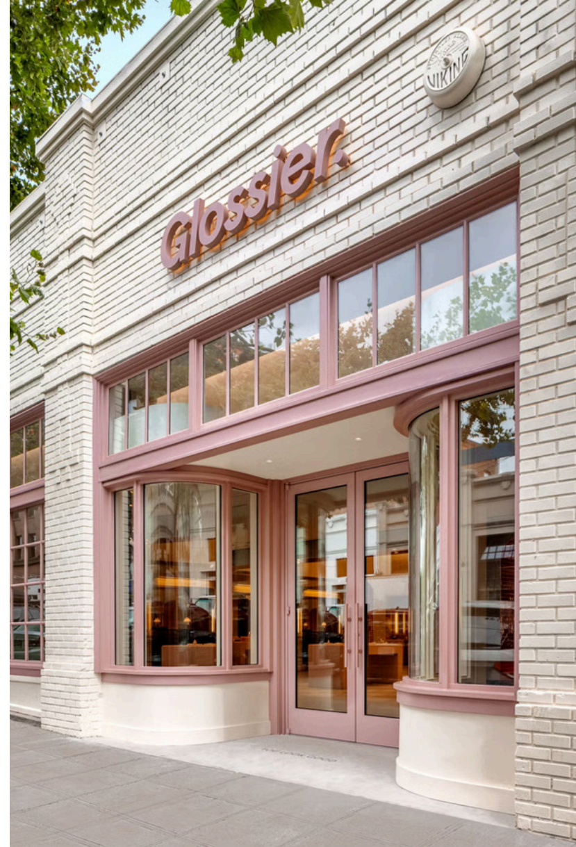
Above: Current Storefront Entrance
