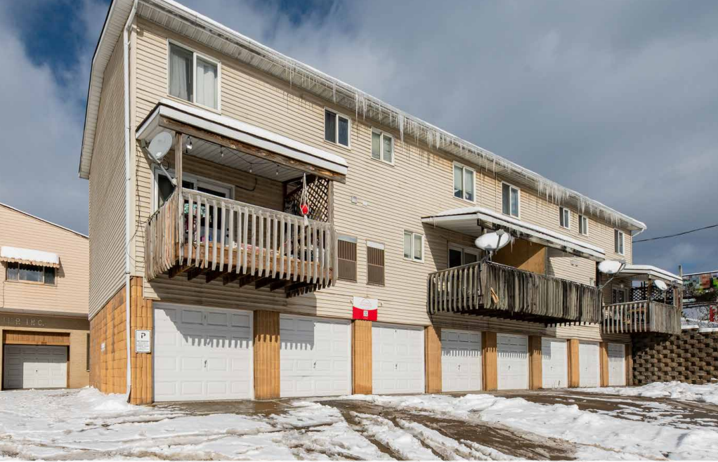
Building A Back Facing Fairmont Road.
