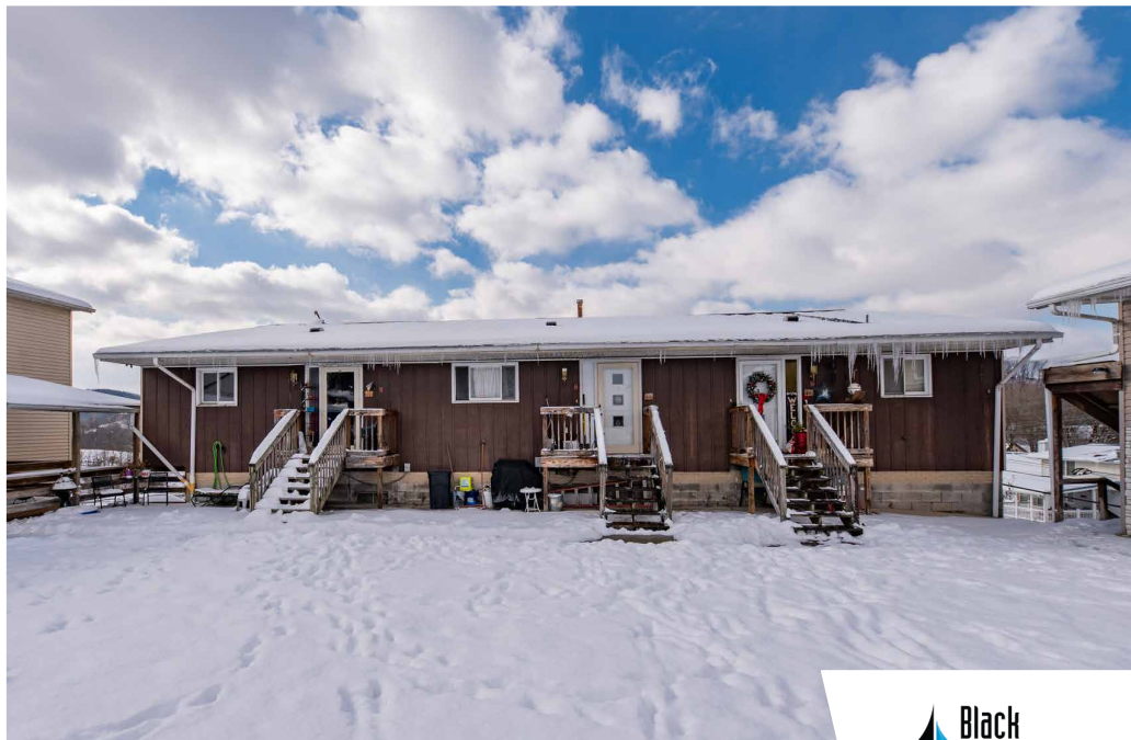
View of Building B from the Courtyard.
