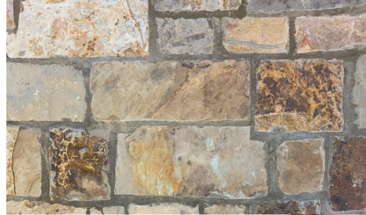
MASONED NATIVE STONE gives the Pendergraft Building its distinctive warmth and durable shape.
