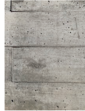
TEXTURIZED CONCRETE SURFACES form walkways and landscaped settings.
