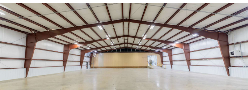
Interior Warehouse Building 2
