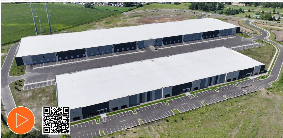
Construction photo, June 2024
