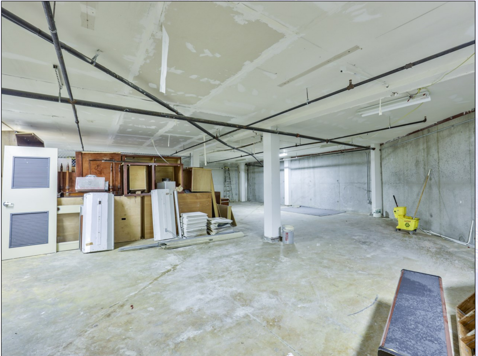
Storage Unit in Lower Level
