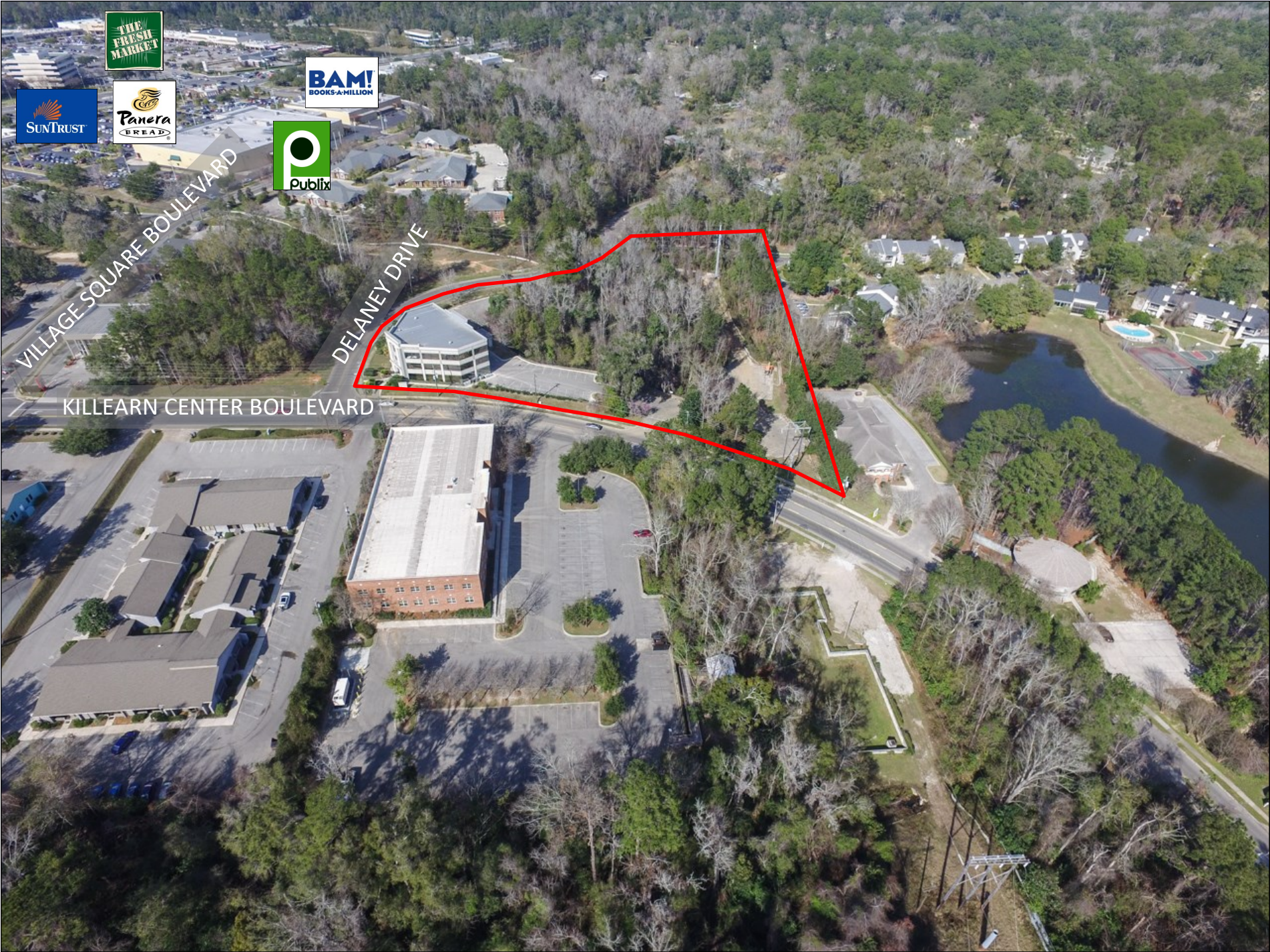
Aerial View Looking North
