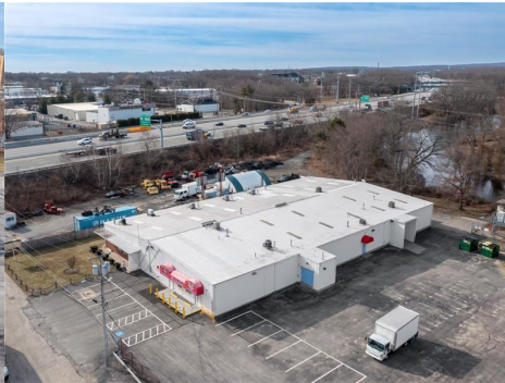
Aerial view with parking
