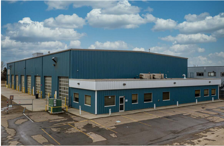
Paved Parking | Heavy Power
