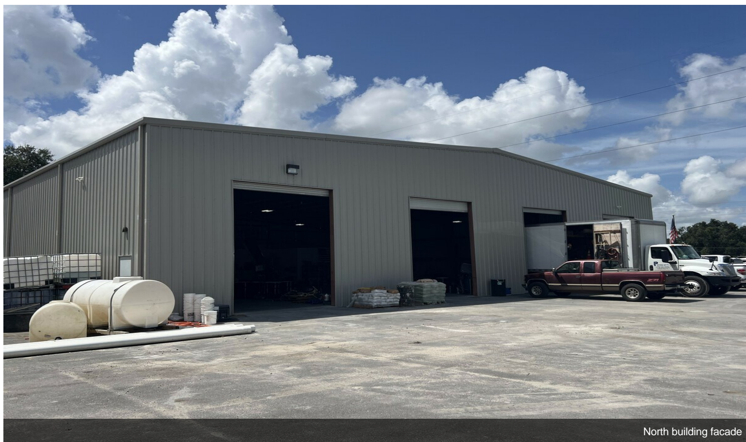
Warehouse and paved parking
