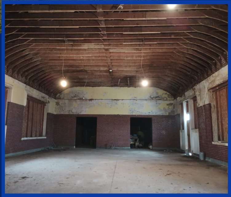
Large Waiting Room with barrel vault ceiling
