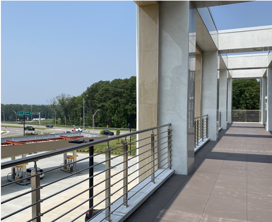
Third floor veranda
