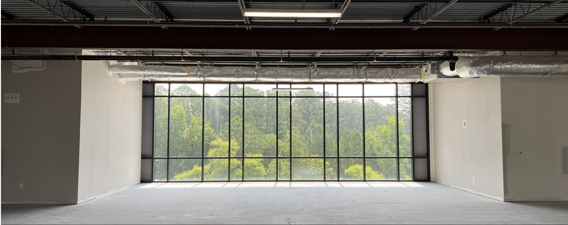
Third floor office
