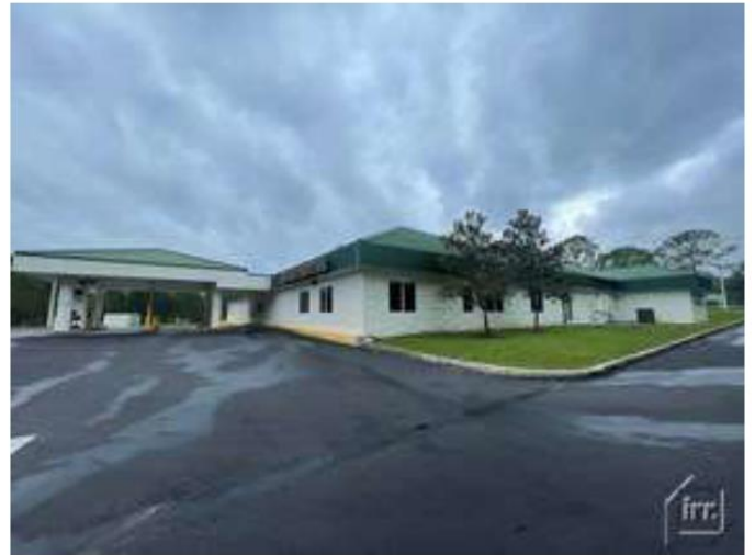
Rear/side/drive-thru lane viewing southwest (Photo Taken on April 7, 2022)
