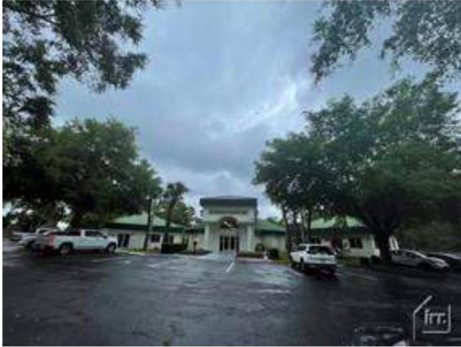
Exterior of subject viewing east (Photo Taken on April 7, 2022)
