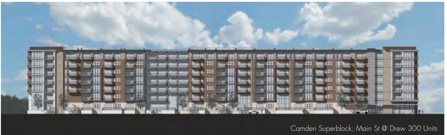
Alliance: Main St @ Alabama 203 Units
