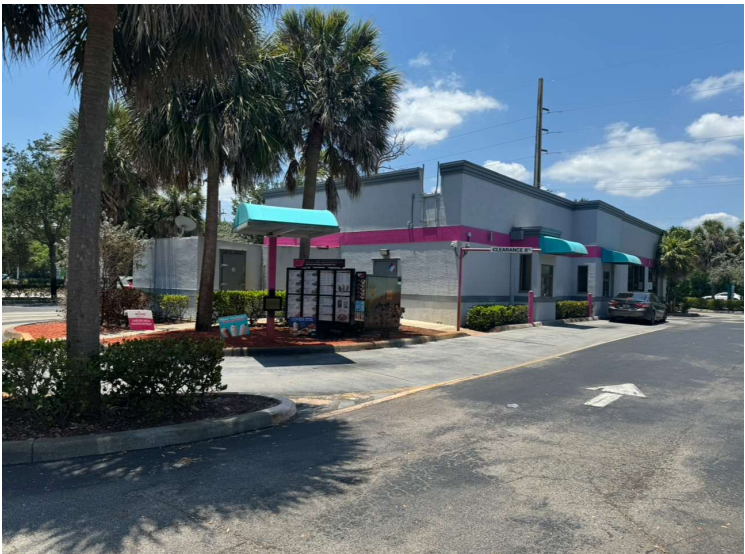
REAR OF BUILDING
