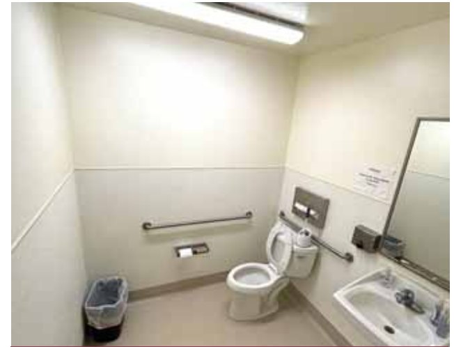
246 Ranch Drive - ADA Restroom
