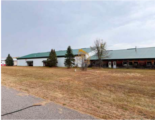
Subject Building - From Edgewater Farm Dr
