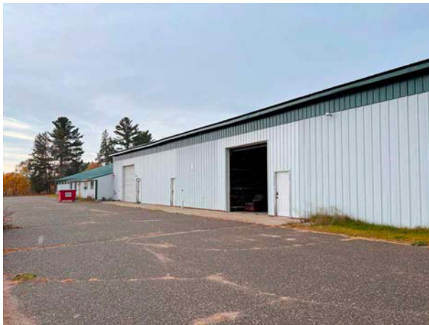
Bay 4 - Entrance & Overhead Door
