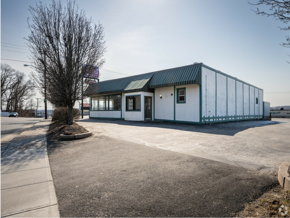
Entrance to 1455 Oaklawn Ave
